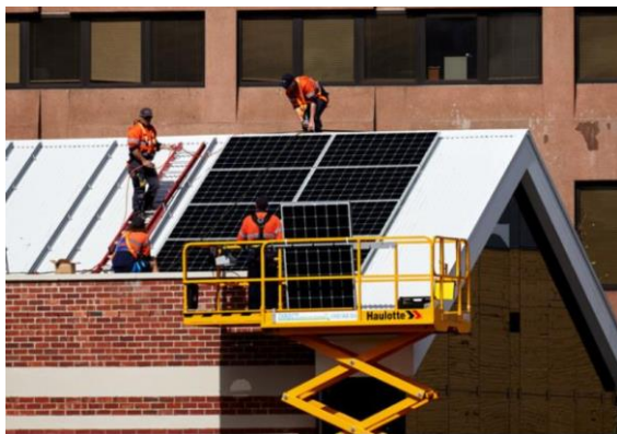
Photo of scissor lift used during installation
